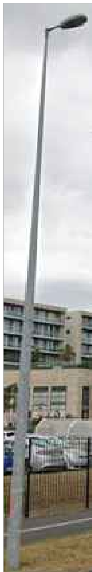
EXISTING COLUMN LIGHTING
